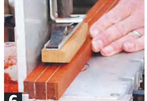
6 Cut a rebate 10 x 7mm on the underside of the timber. It's easiest to do this on a router table with a straight bit
